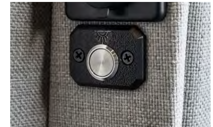
Figure 5-9. Ceiling Lights Push Button
